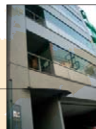
OPTIS Headquarters Toulon, France
